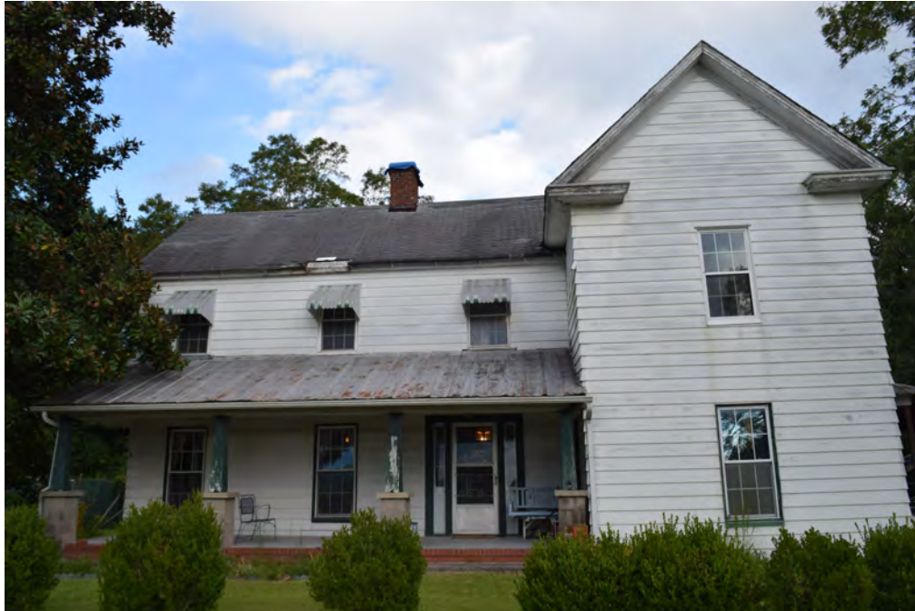
Humphrey-Armstrong House facade, view to the northeast
