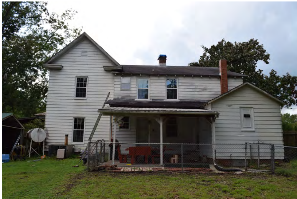
Rear elevation, view to the west
