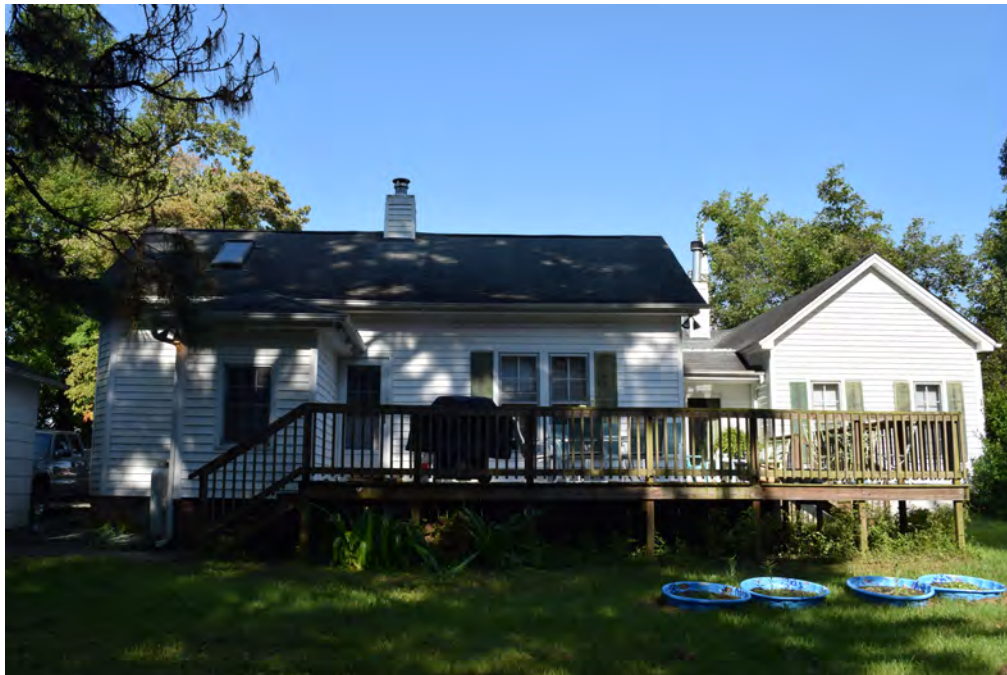
Rear elevation, view to the east (former kitchen in the foreground)
