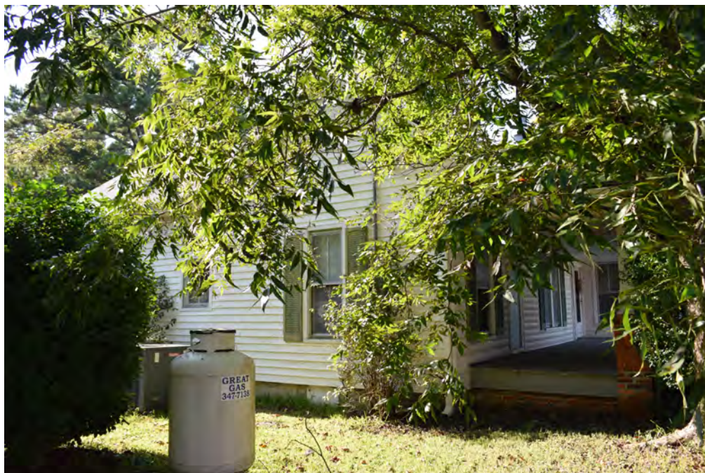
Southeast (front) corner of the Nick and Ella Burton House, view to the northwest
