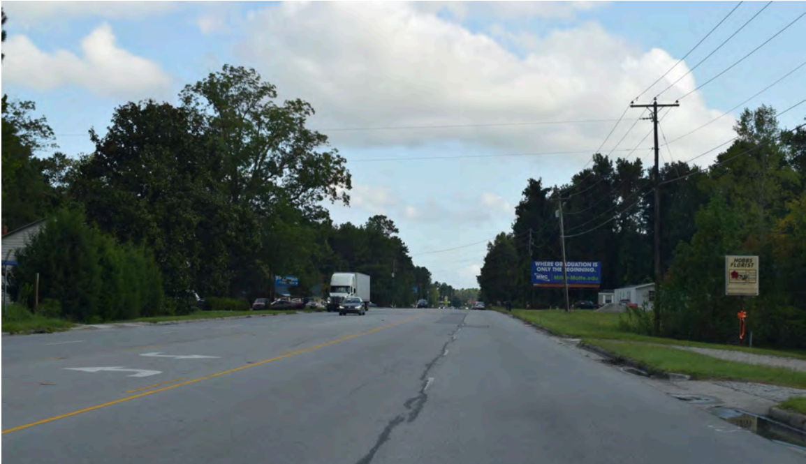
Project area on US 258, view to the south toward Blue Top Road
