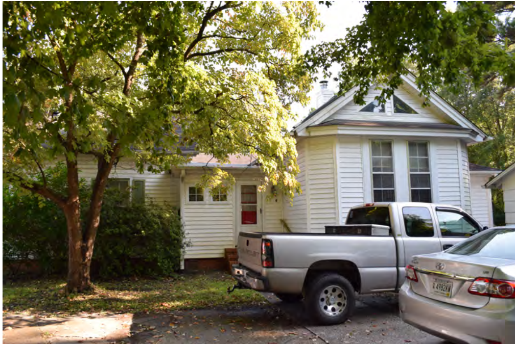
North elevation, former detached kitchen to the right, view to the south
